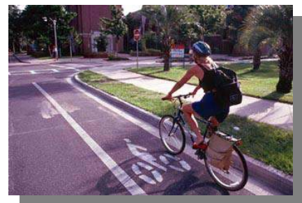
Figure 3.3. Bicycle Lane. Source: www.pedbikeimages.org
