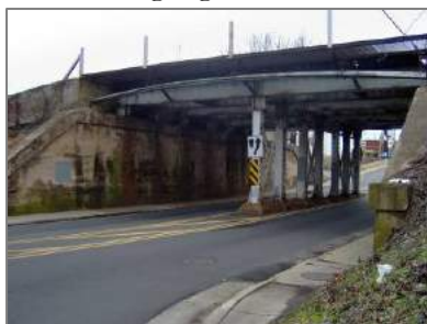
Figure 3.10. Tate Street underpass
