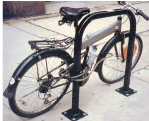
Figure 5.1. Inverted-U Style Bike Rack. Source: APBP Bike Parking Guidelines
