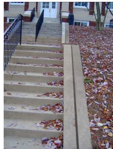
Figure 4.18. Stair channel (Brown Building photo).
