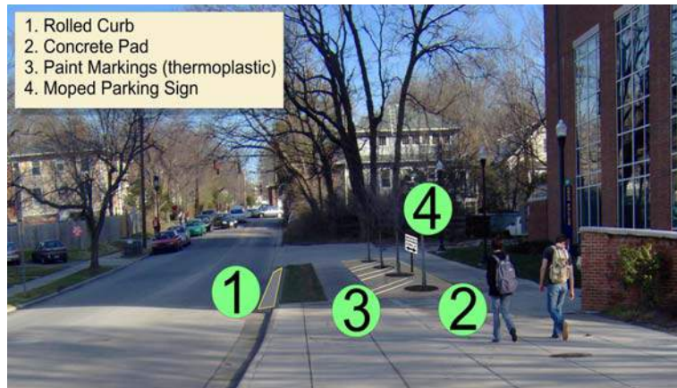
Figure 5.13. Proposed “moped only” parking area for UNCG. Located along Carr Street in front of the Sullivan Science Building.
